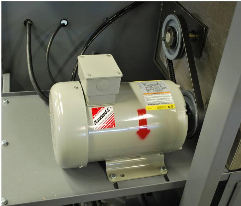
Figure 14 - Main Blower Motor with Direction Indicator
