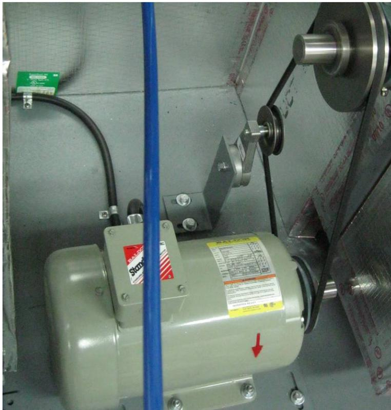
Figure 2 - Blower Motor with Direction Indicator
